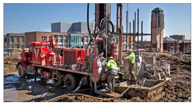
Figure 05. Geothermal drilling on Hayward Street
